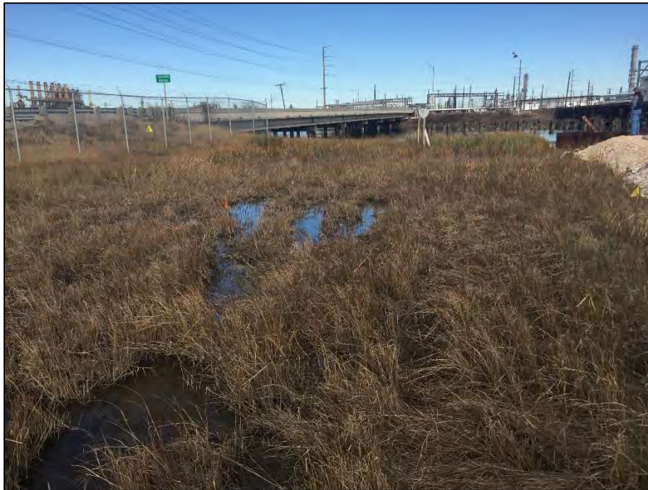
PHOTO 2 Remaining Tidal Marsh Looking North
