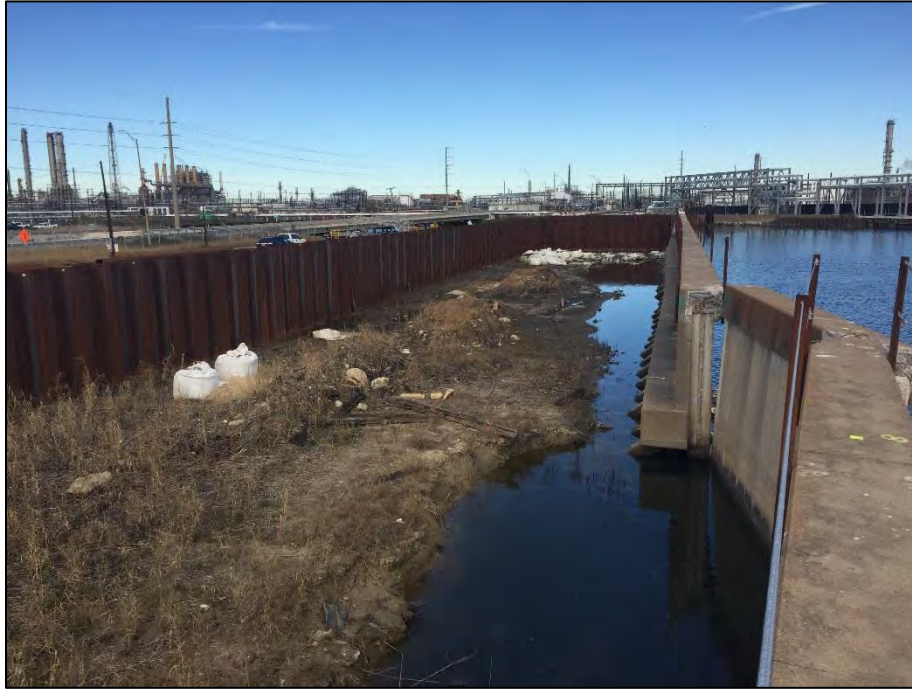
PHOTO 5 Inside Sheet Pile Containment
